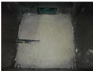
The initial state of inside of the furnace
